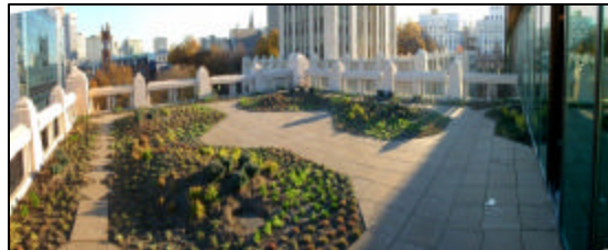
Green Roof in Atlanta GA
