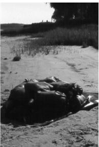
Figure 11.2. Barrel well stabilized with Geo Fabric<sup>TM</sup> and sandbags. (SCIAA)
