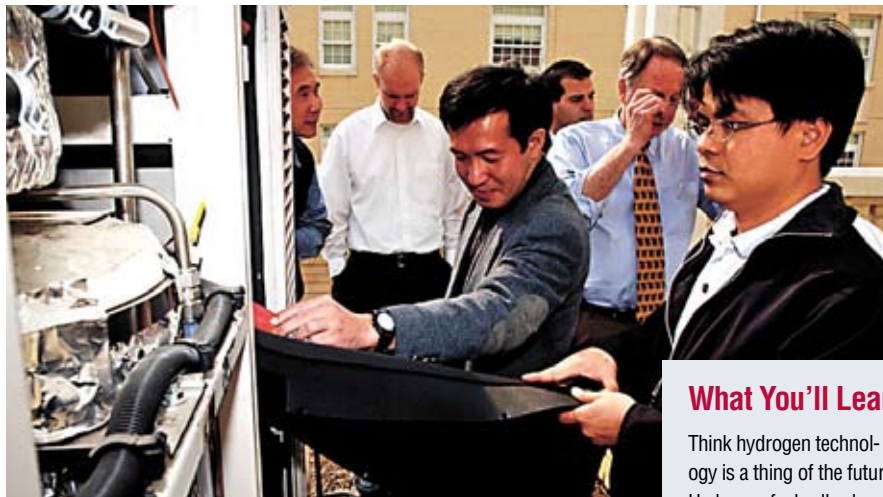
Chemical engineering students Masato Ohasi, left, and Konalayutt Punyawudho check out the hydrogen fuel cell next to the West Quad dormitory. Electricity and hot water for the dorm are generated partly by the fuel cell. Photo by Jeff Blake The State .
